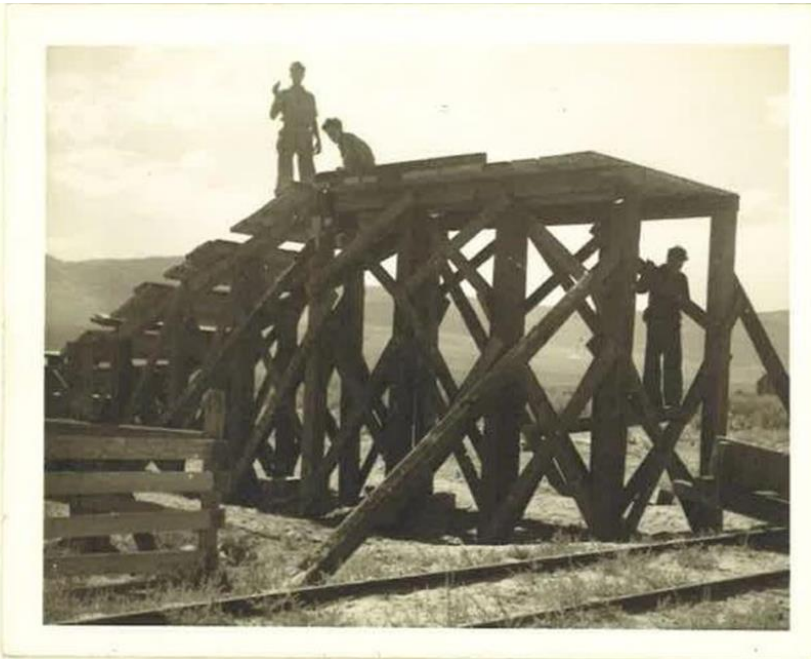
14. Building our loading dock at Benton Station, using second hand timbers purchased in an L.A. wrecking yard with the proceeds from the initial tailings shipment. The ramp is a steep 10% grade dependent, unfortunately, on the advice of the truck driver. It was no go. The loaded truck was waiting, the scraper loader was idle back at the meadow, our train of gondolas stood empty with demurrage charges looming- it was time for radical action.
