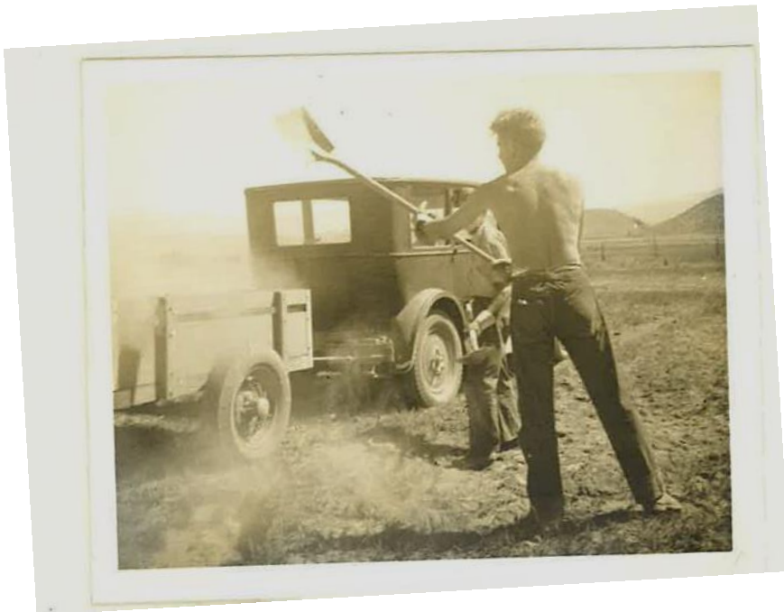
10. both the Dodge and the prospectors pressed into service to haul the initial shipment of tailings to Benton Station. The tailings had been repeatedly ground in the old stamp mill in a vain attempt to break out the values, so we had to deal with a dust that was as fine as flour and as red as rust.
