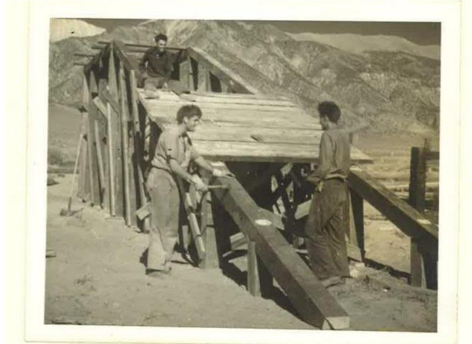
15. After a long night of work, the loading platform was lowered by three feet, extended an illegal two feet closer to the tracks of the siding, and the ramp brought down to a grade feasible for the dump truck. Here in the morning Johnny Allingham, Earl Williams and Pierce Clarke nail down the las of the flooring plank
